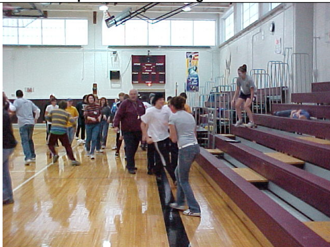
Photo 3 – Shortly After Bleacher Collapse
