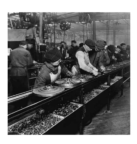
These people work on an assembly line at Ford Motor Company. In 1913 American automobile pioneer Henry Ford instituted the assembly line process, in which each worker performs only one specialized task, in order to speed production.
