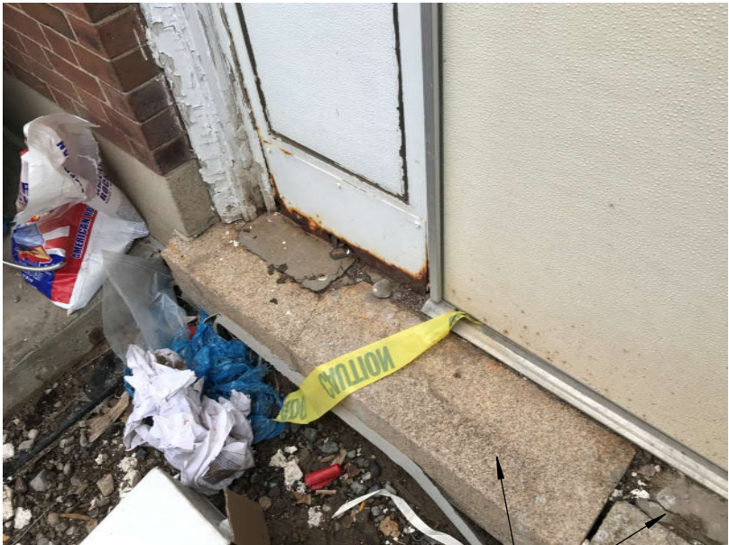
REMOVE EXISTING CRACKED THRESHOLD AND CONCRETE INFILL PATCHES - FULL WIDTH OF MASONRY OPENING
